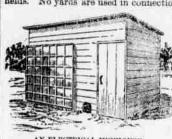
AN ELECTRICAL HENHOUSE. with them, and they are set eight rods distant from each other, allowing about 100 hens to the acre. By means of an improved feedbox any number of flocks can be fed simultaneously, each in its own house, by simply pressing an elec-tric button. The doors can be opened or closed in the same way.
