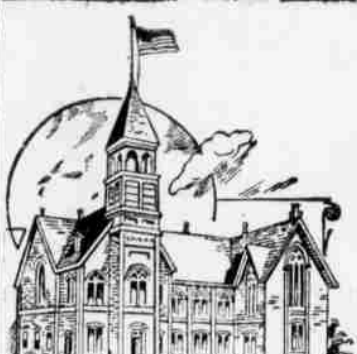
State Normal School building.
