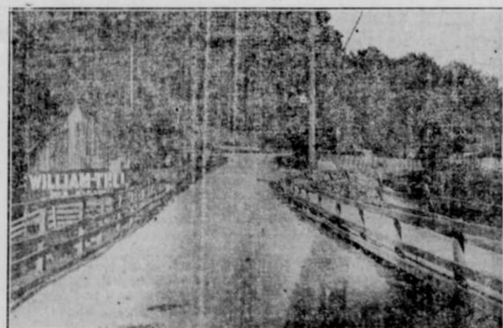
Same Road After Improvement.
