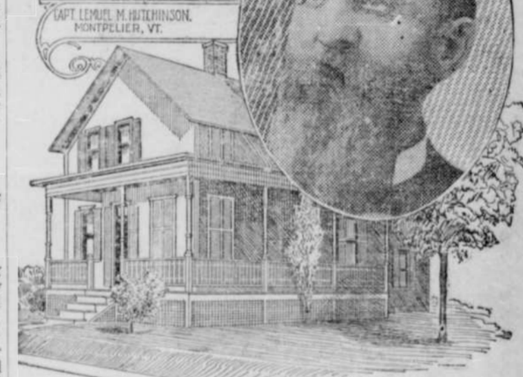
The Home of Captain Hutchinson, of Montpelier, Vt.
