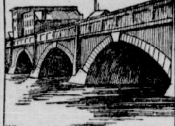
STEEL-CONCRETE BRIDGE, PLAINWELL, MICH.
