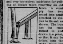
drawn to a point, so that it can be driven into the stake, when the latter can be STAKE PULLER. pulled up with ase. If the stake is large the arms can easily be sprung apart so that the
