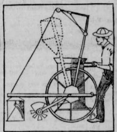
STREET SWEEPER IN OPERATION.
