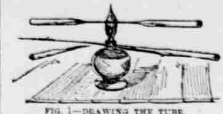
FIG. 1.—DRAWING THE TUBE.
