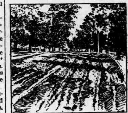
ROAD READY FOR OILING.
