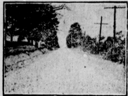
A WELL BUILT CONCRETE ROAD. [From Good Roads Magazine, New York.]
