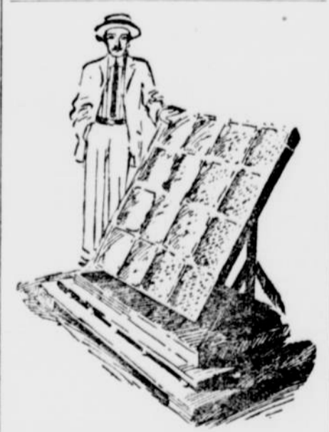
LOW POWER GENERATOR.
