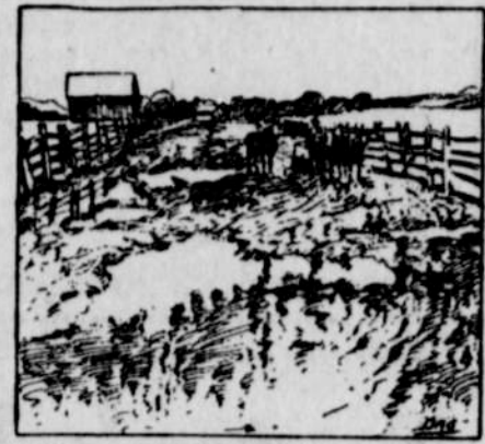
TYPICAL CLAY ROAD BEFORE IMPROVEMENT.
