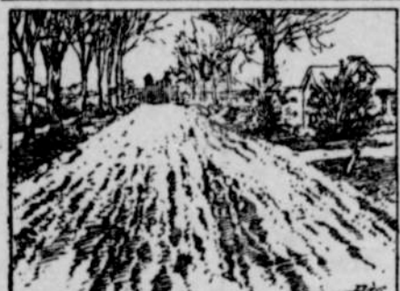
OLD ROADMAKING METHOD RESULTS IN EITHER A MUD OR DUST ROADBED.
