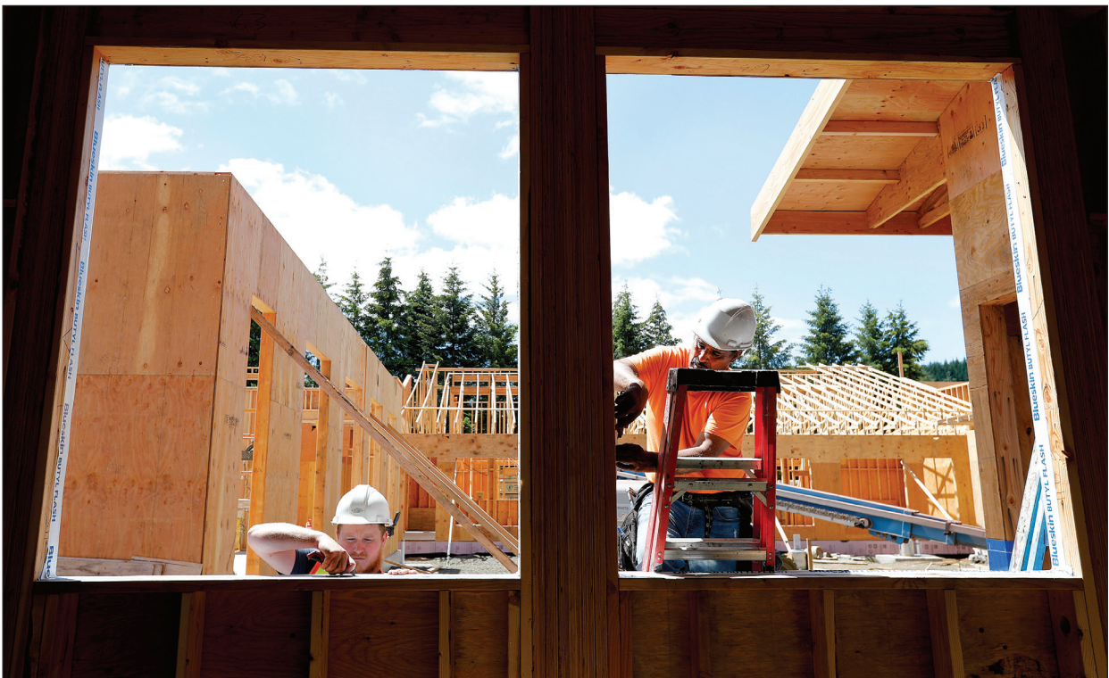
Huri Scherbakob, left, and Javier Mota, both siders with Bold Elements of Woodburn, apply an air, water and moisture vapor barrier to a window while working on the child development center under construction on the Tribal campus on Tuesday, June 18.
