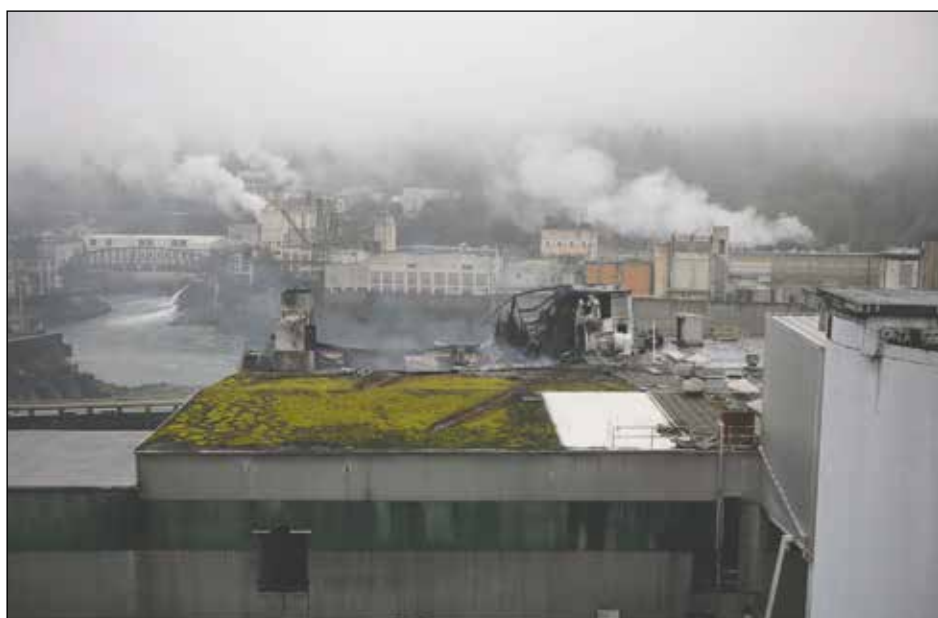
Smoke rises from one of the buildings on the Tribally owned Blue Heron Paper Mill site on Sunday, Dec. 6.
