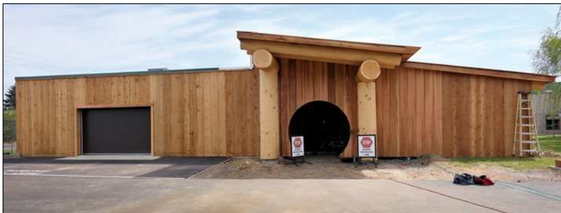
Chachalu Tribal Museum & Cultural Center Phase Two construction includes a newly designed entryway to the building.
