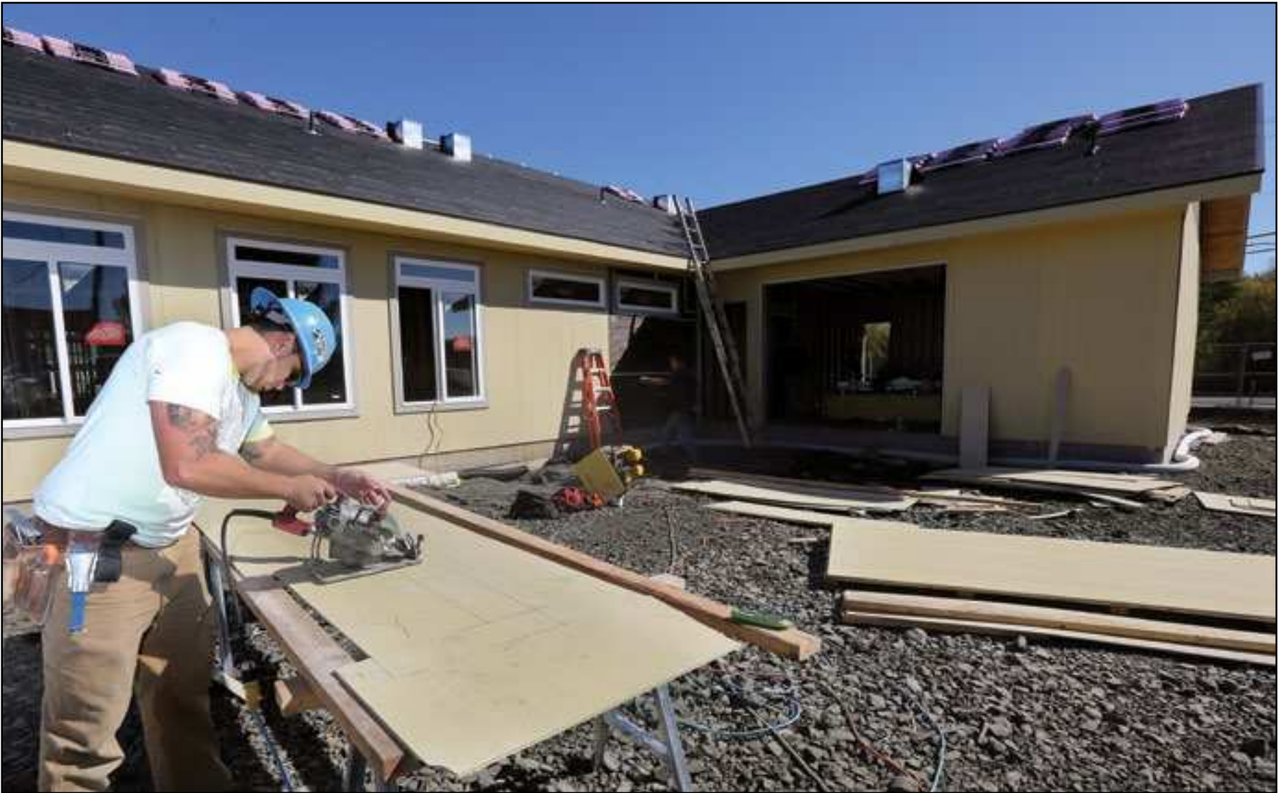
Jordan Tinoco cuts siding for the new Grand Ronde Tribal Police Station as construction continues on Friday, Sept. 9. The 4,400-square-foot building is expected to be completed by Dec. 1. Funding for the $1.1 million building includes a $500,000 Housing and Urban Development Indian Community Development block grant, $167,000 in HUD Indian Housing block grant funding and some Tribal funds. Cearley Construction, located in Estacada, is the contractor for the job and is a Tribal Employment Rights Ordinance-certified Indian-owned business. Tinoco is a Tribal member working through the Tribe's TERO office.
