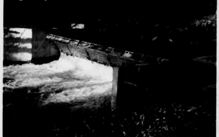
Agency Creek Fish Weir
