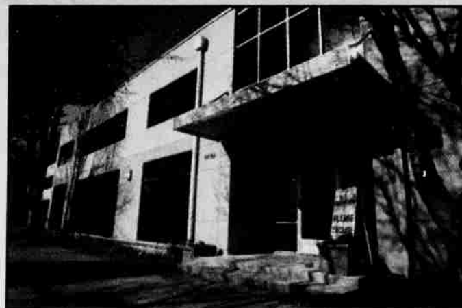
The new Portland satellite office building is located at 4445 S.W. Barbur Blvd., Portland.
