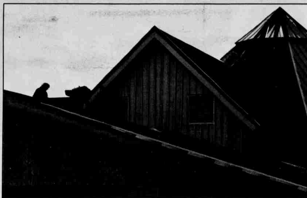
Roofing work continues on the Tribal Health & Wellness Center expansion on Wednesday, Jan. 27. The expansion should be completed in March.
