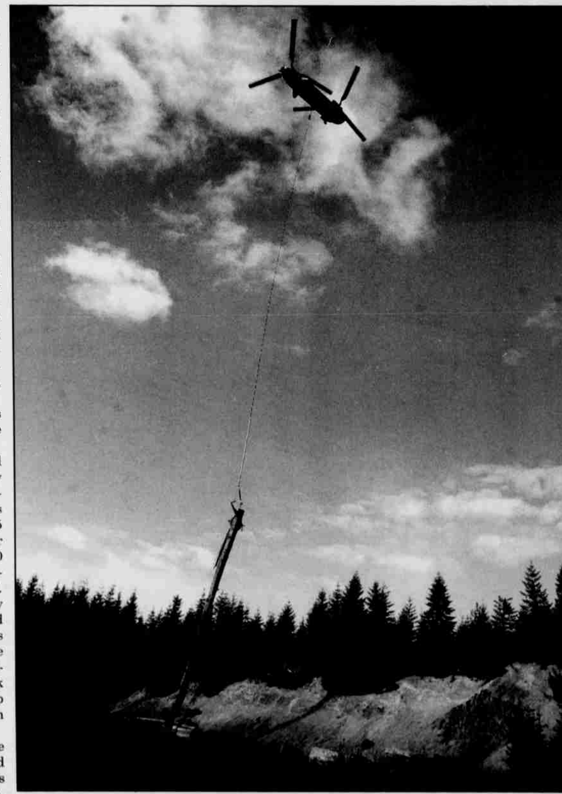
A Chinook helicopter lowers a cedar log to the landing site off Soda Fork Road. The U.S. Forest Service is providing the wood to the Grand Ronde Tribe for a longhouse that is planned to be built using traditional methods.
