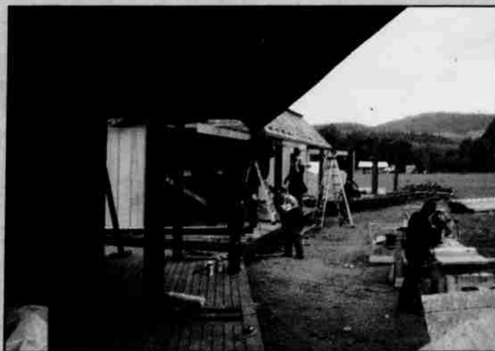
Tribal members from the Tribe's pre-apprenticeship program work on the Elders' seating area at the new pow-wow grounds.
