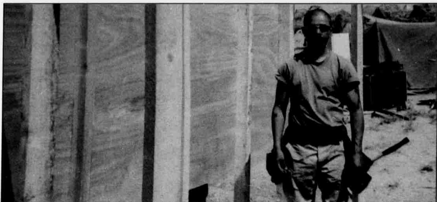
Hostler, with the 52nd Engineers in Mosul, Iraq, where the unit built shelter for other GIs.
