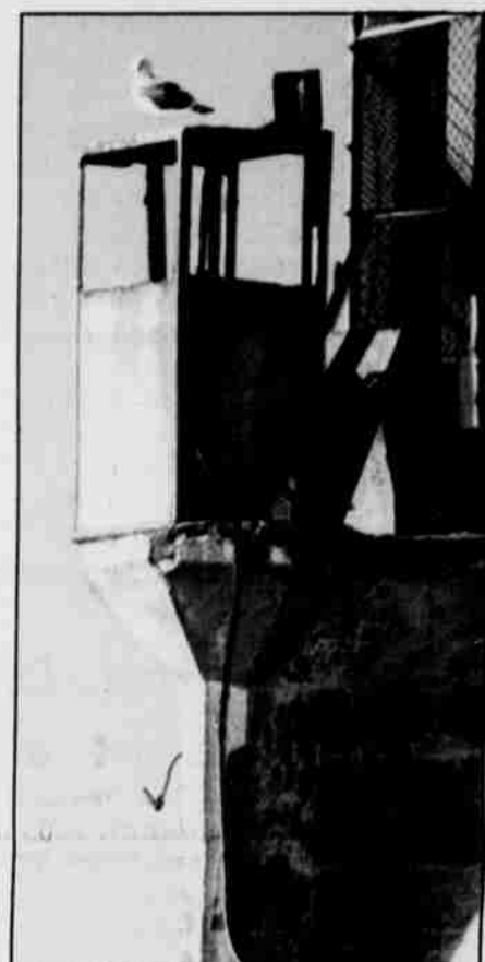
Guard Tower on Alcatraz
