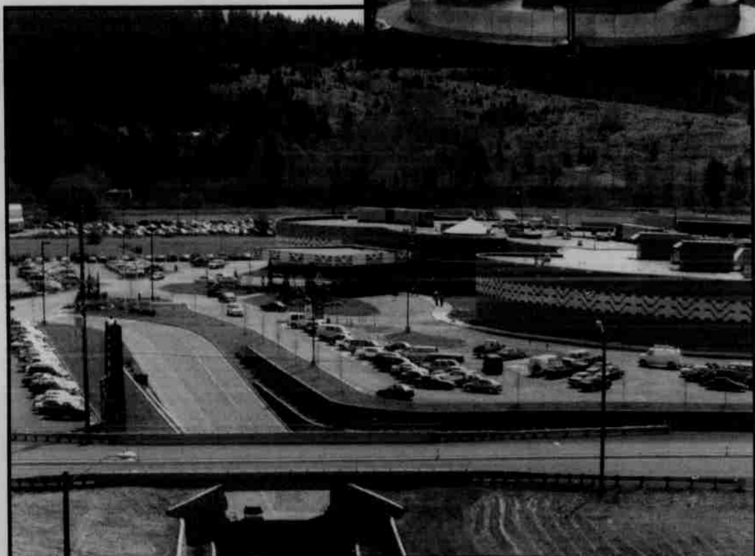
Tribe builds highway underpass to ease local traffic.
