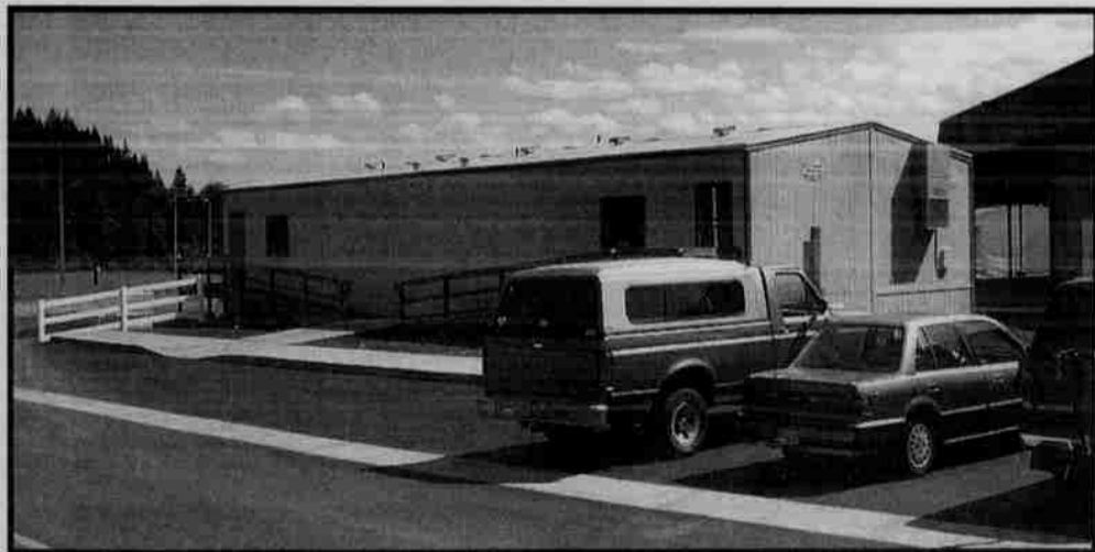
The Tribe's new Before & After Care building sits directly behind Grand Ronde Elementary School. This new modular gives the program much needed space.
