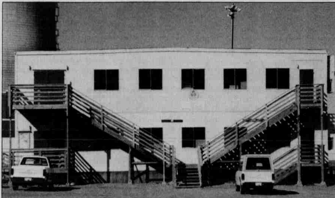
The new modular building will provide training facilities and office space for several tribal departments that have been expanding.
