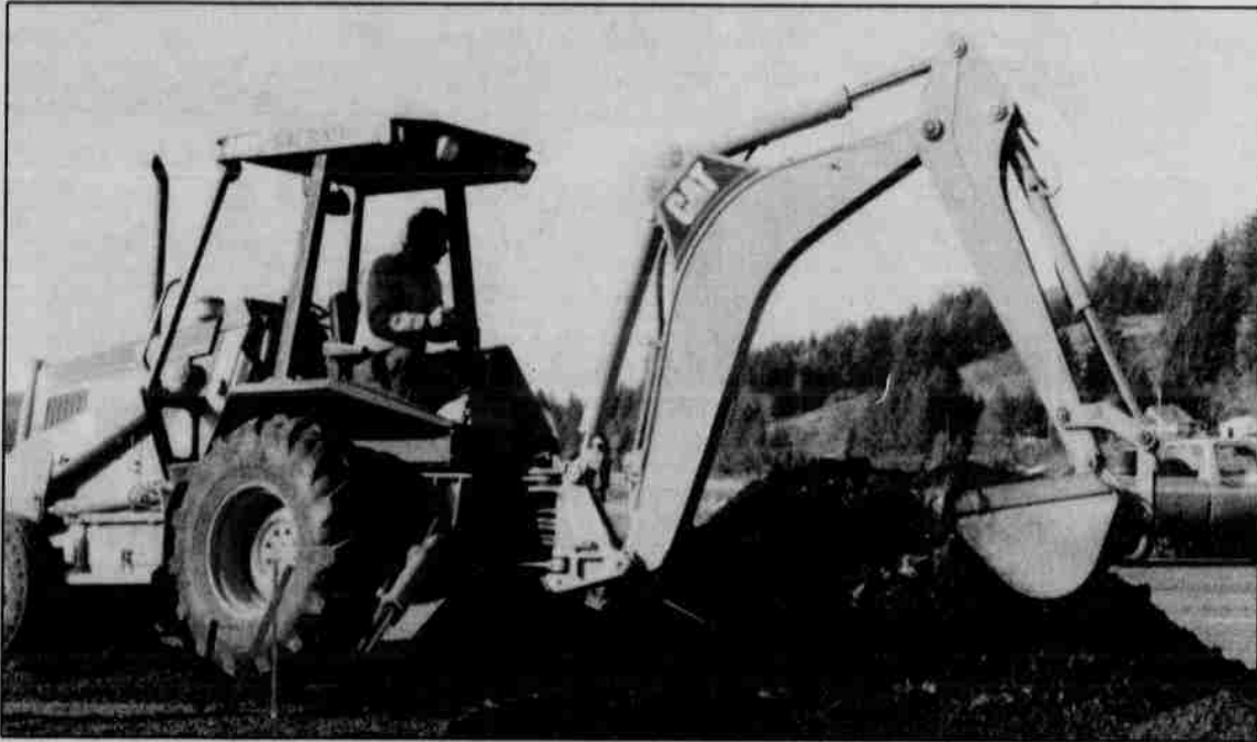
Construction worker digging footings for gaming center's concrete foundation.
