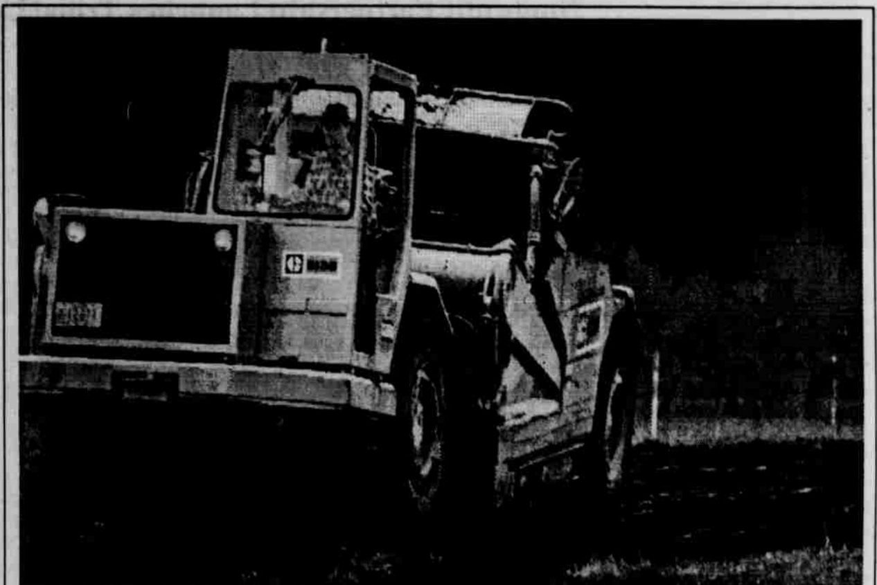
This scraper is working to put in the road that will lead to the new Tribal office complex on Grand Ronde Road approximately one mile north of the Tribes' current office in the old manor. Tribal chairman Mark Mercier would like to ask for everyone's patience during the move which should be complete some time in December.
