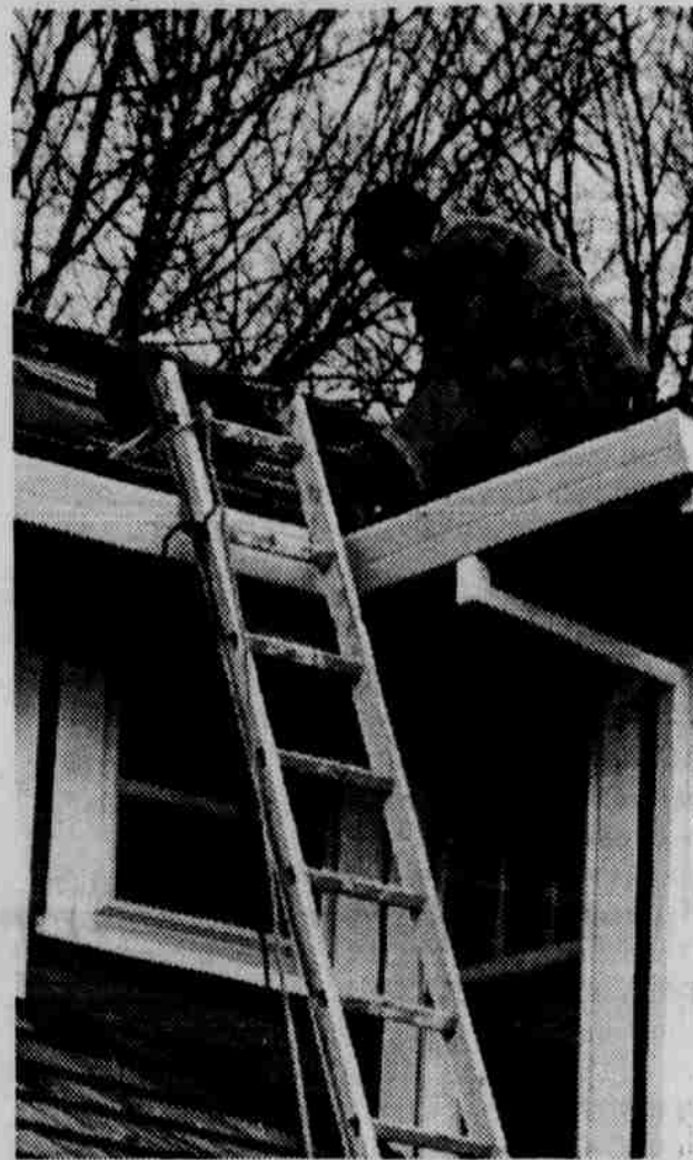
Mark Grosser got the job of repairing the Depot roof.
