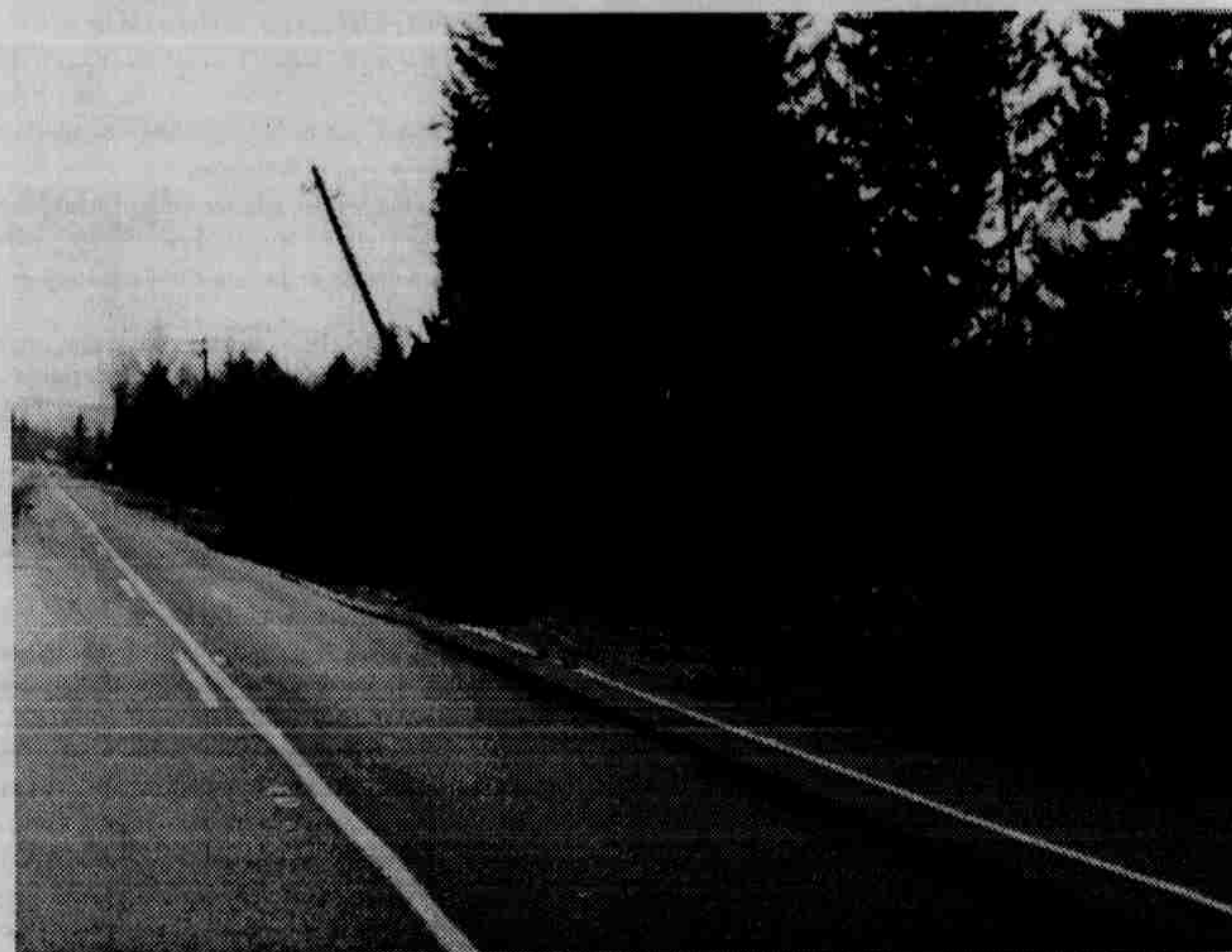
The high winds caused considerable damage all along Highway 22. Powerlines were knocked over by falling trees.
