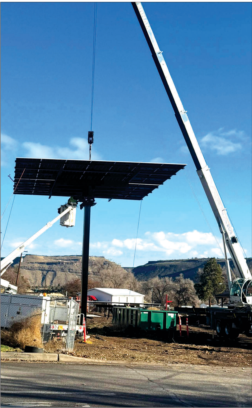
Solar Stacker installation outside the Commissary business center.
