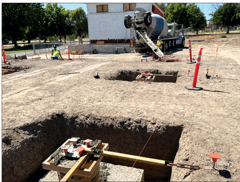
Construction workers on site at the food court area.
