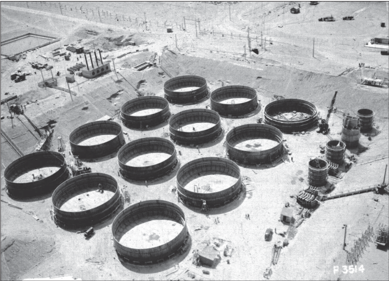
Nuclear waste tanks, built early in Hanford's development.
