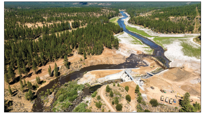
Area of Klamath River where dam was breached.
