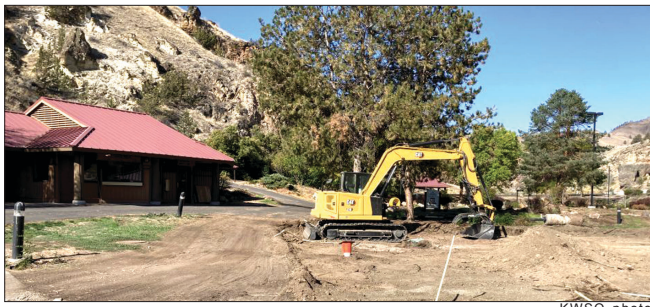
March construction work at Kah-Nee-Ta Resort & Spa.
