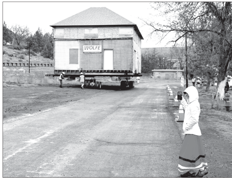
People stopped to take pictures in April of the Commissary building in transport to its new location by the highway.
