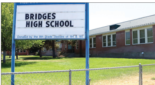
Bridges High School work is under way.
