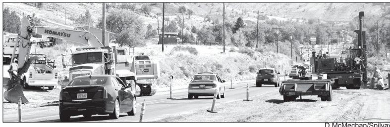
View toward casino and museum, sidewalk work on the right.
