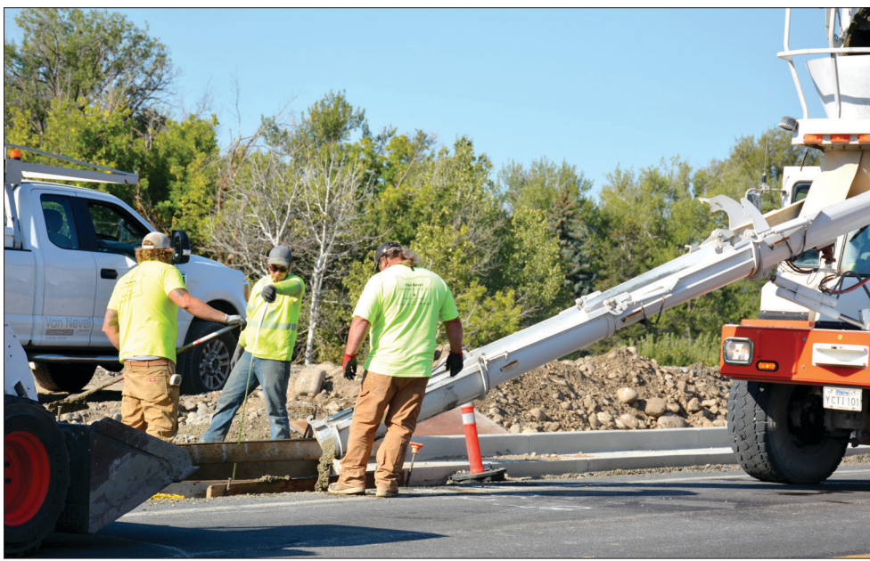
Construction crew pours concrete for the new pedestrian path along Highway 26.
