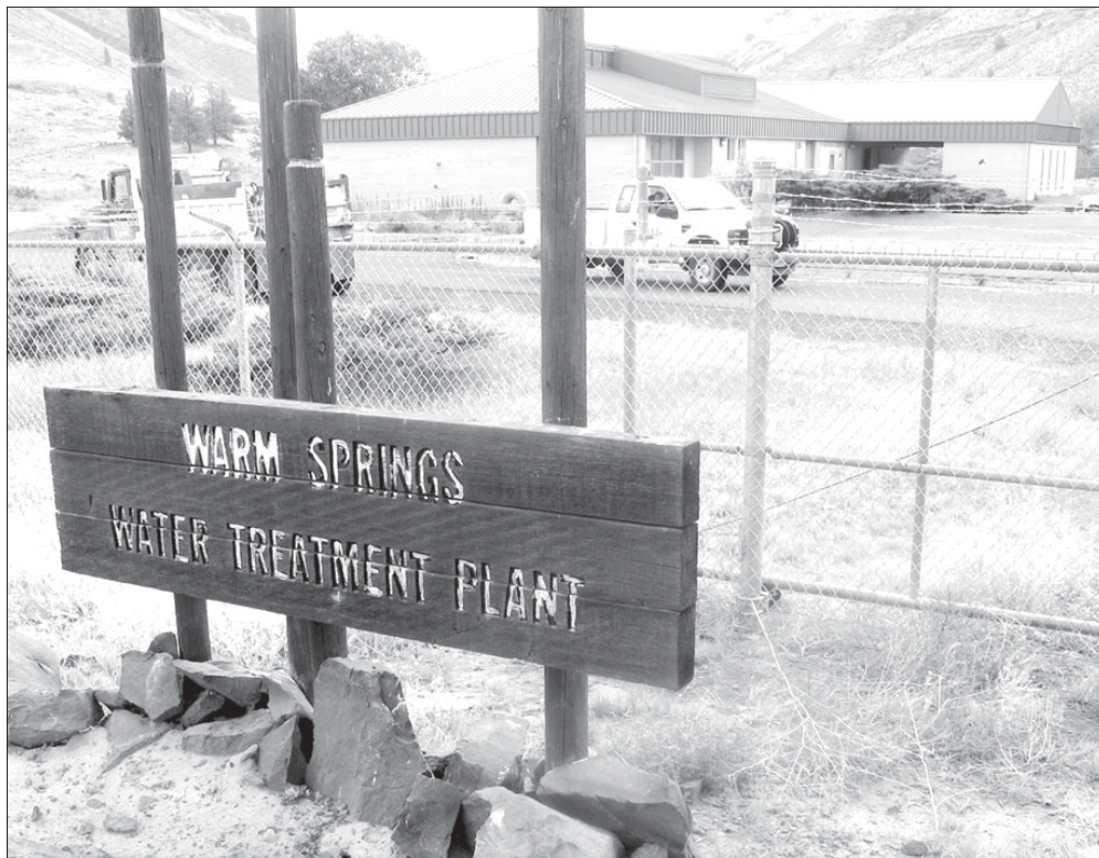
Estimated cost of replacing the treatment plant is at least $20 million.
