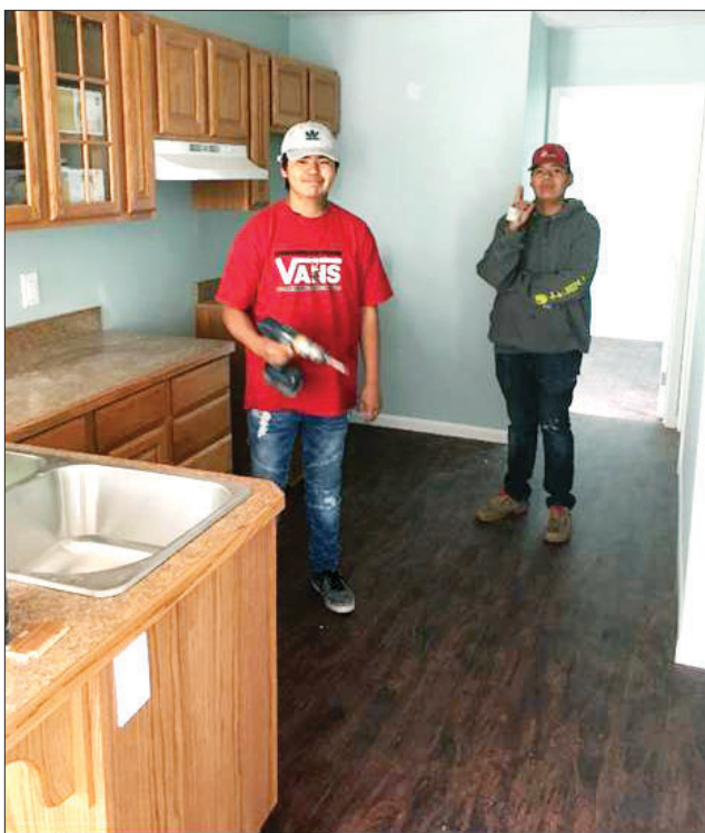
Roots students at the renovated veterans trailer. Courtesy photo.
