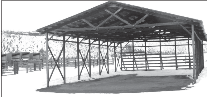
Existing structures at the tribes' Schoenhagen property.
