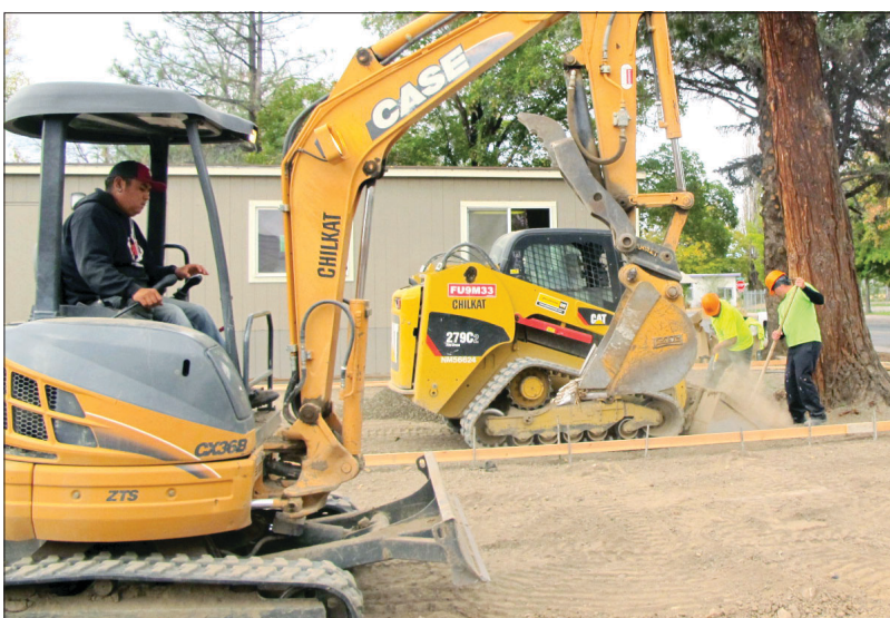
Construction works on the landscaping at the front of the building.
