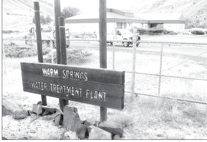
The treatment plant on the Deschutes River.
