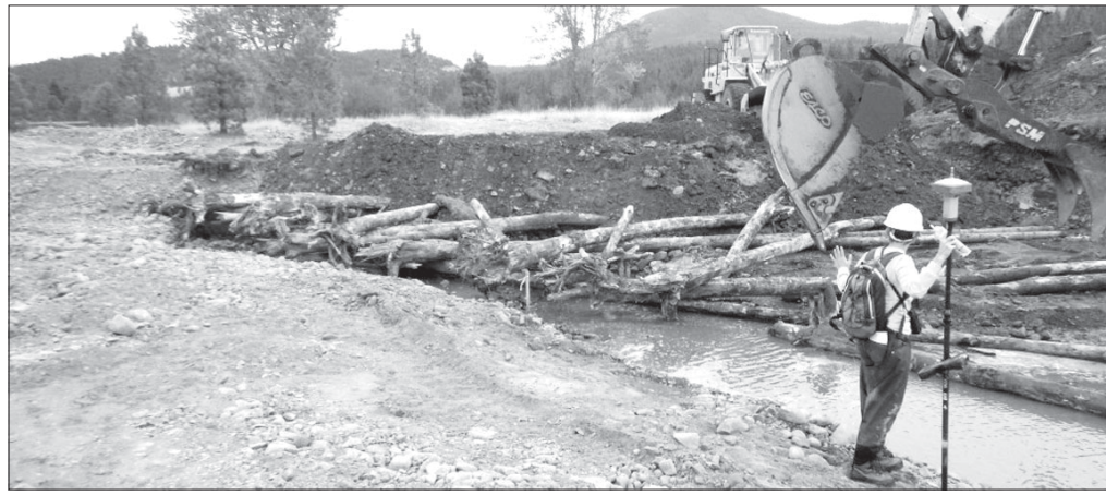
Creating in-stream features, during phase 4 of the project.
