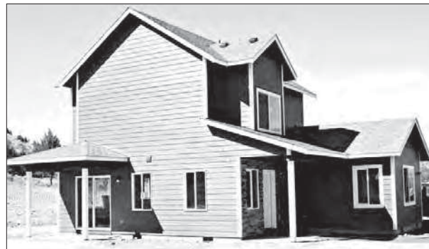
One of the new units at Greeley Heights.
