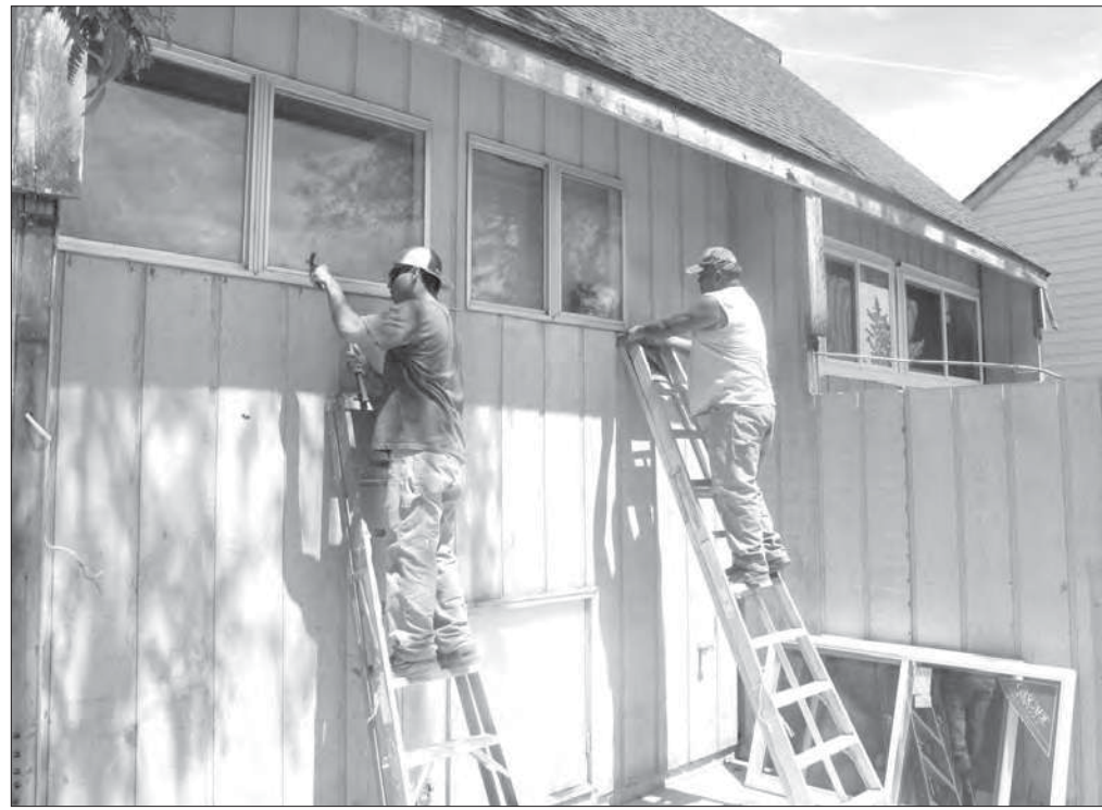
Albert Adams and Elmer Charley remove the old windows from the Tenino Apartments.
