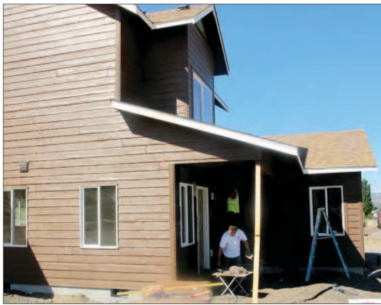
New Greeley Heights unit nearing completion. Dave McMechan/Spilyay
