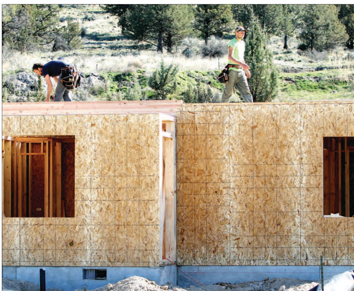
One of the units under construction.
